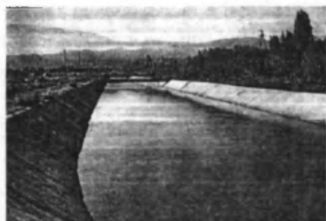
59-rasm. Yaxlit beton to'shamali kanal.
